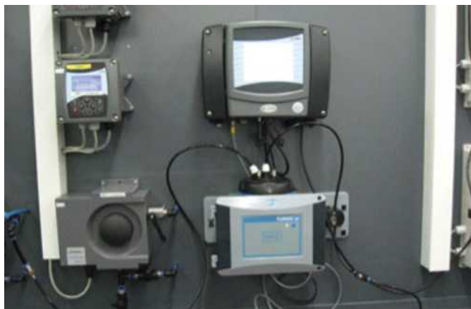
Figure 3: TU5400 with SC1000 installation in a German drinking water plant
