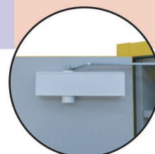
Self-closing door(s) with thermo-fuse
