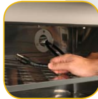
Interior Access Port
